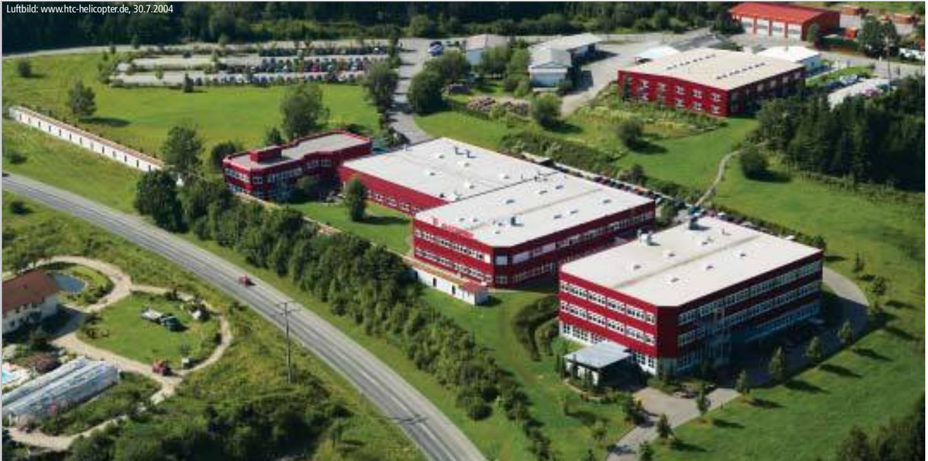
TR-Electronic, in the foreground the 200m laser referencing track (white). Behind, on the hill, TR-Systemtechnik
